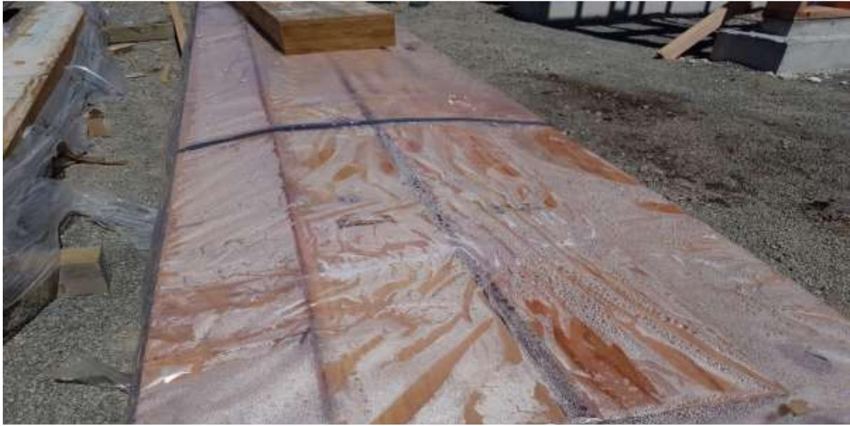
This timber was saturated within the packaging and went on to form mould within the new home prior to lining. This illustrates the moisture issues encountered during the current process from treatment plant to suppliers yard through to delivery on site.
