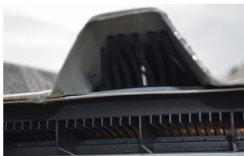
Fig D: VENT Over Fascia Vent G1200N fitted with VENT Eaves Comb Filler G1275
